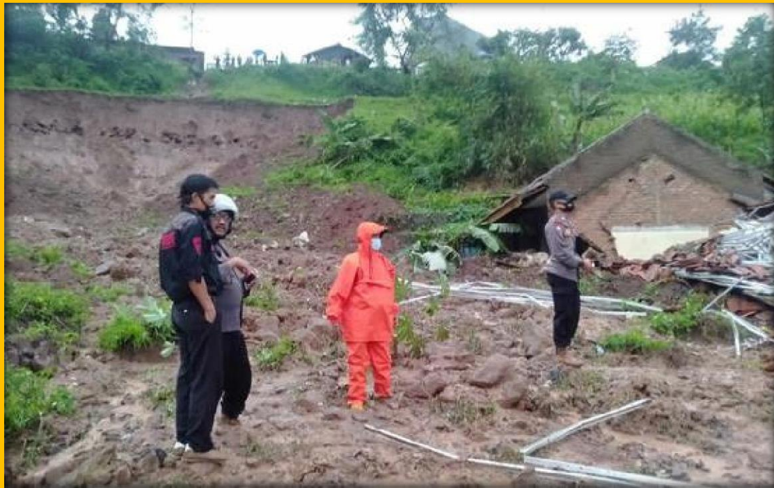
After First Landslide
