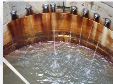
Large diameter drainage well at Yachi landslide area of Akita
