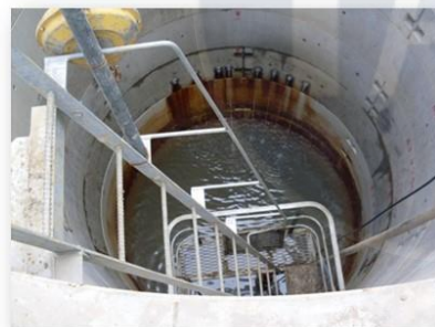
Large diameter drainage well at Yachi landslide area of Akita
