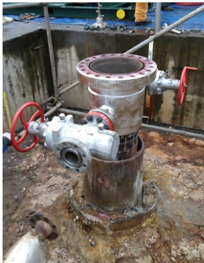
Master Valve Change using Packer
