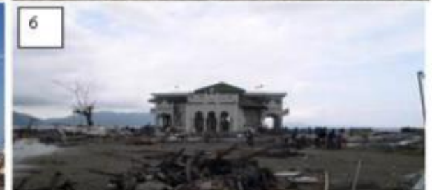
Figure 4 Typical damage to different types of houses due to tsunami with different flow depths in Banda Aceh and Nias Island after the 26 December 2004 event. Most of the 3 storey reinforced concrete structures survived the tsunami with flow depths greater than 10m (photo 5 and 6) whereas other buildings which surrounded these were completely wiped out. With this flow depth, no sheltering effects from the buildings or trees reduced the tsunami impact. A simple house with a palm tree roof was resistant to the earthquake shaking (photo 1) when compared to the neighbouring concrete house (photo 2). However, this house suffered damage from the tsunami with a flow depth of 1.8 m or half of the height of the house (Modified from: Prasetya et al. 2008).
