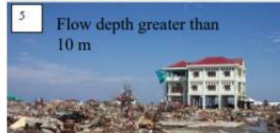
Figure 4 Typical damage to different types of houses due to tsunami with different flow depths in Banda Aceh and Nias Island after the 26 December 2004 event. Most of the 3 storey reinforced concrete structures survived the tsunami with flow depths greater than 10m (photo 5 and 6) whereas other buildings which surrounded these were completely wiped out. With this flow depth, no sheltering effects from the buildings or trees reduced the tsunami impact. A simple house with a palm tree roof was resistant to the earthquake shaking (photo 1) when compared to the neighbouring concrete house (photo 2). However, this house suffered damage from the tsunami with a flow depth of 1.8 m or half of the height of the house (Modified from: Prasetya et al. 2008).
