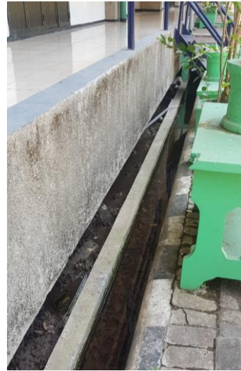
Elevated Structure Departemen Kimia ITS
