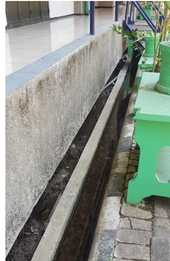
Elevated Structure Departemen Kimia ITS
