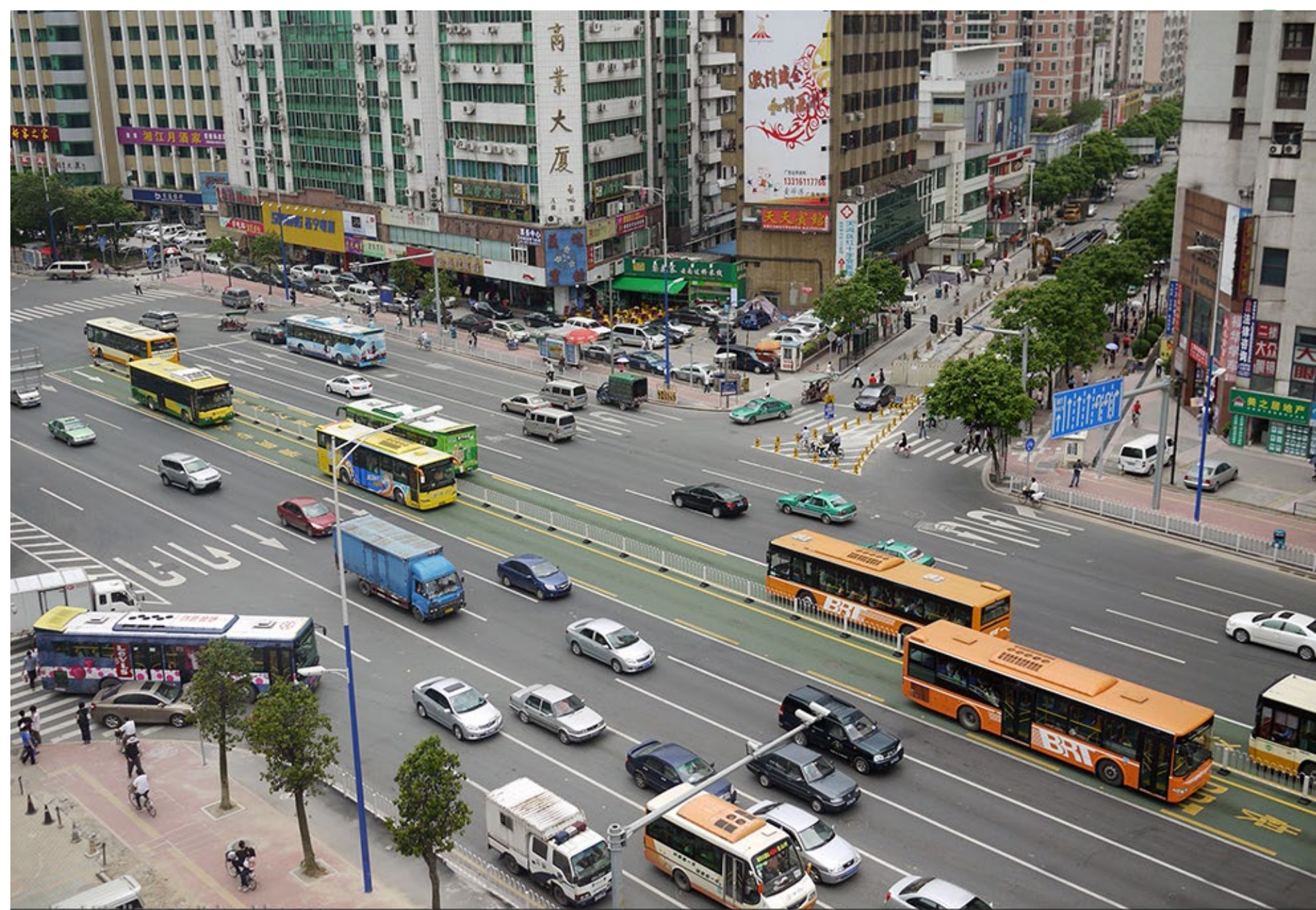
Changed to a 2-phase intersection and combined with at-grade BRT station access. Previously a major traffic blackspot, now operates smoothly
