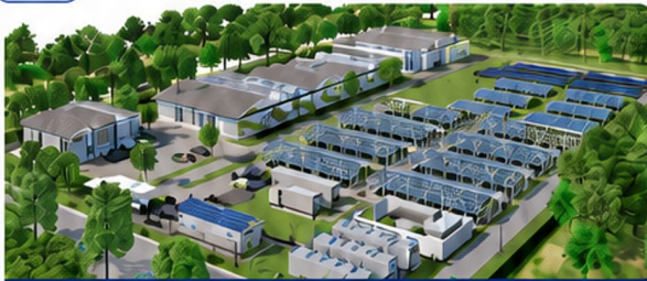
Fasilitas REIDI (Renewable Energy Integration Demonstrator of Indonesia)
