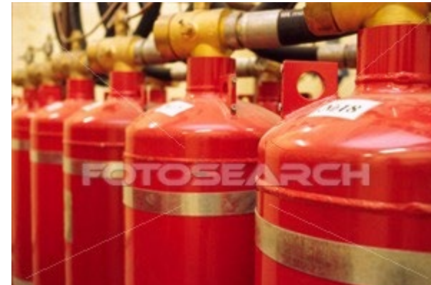
Fire fighting system filled with inert gas
