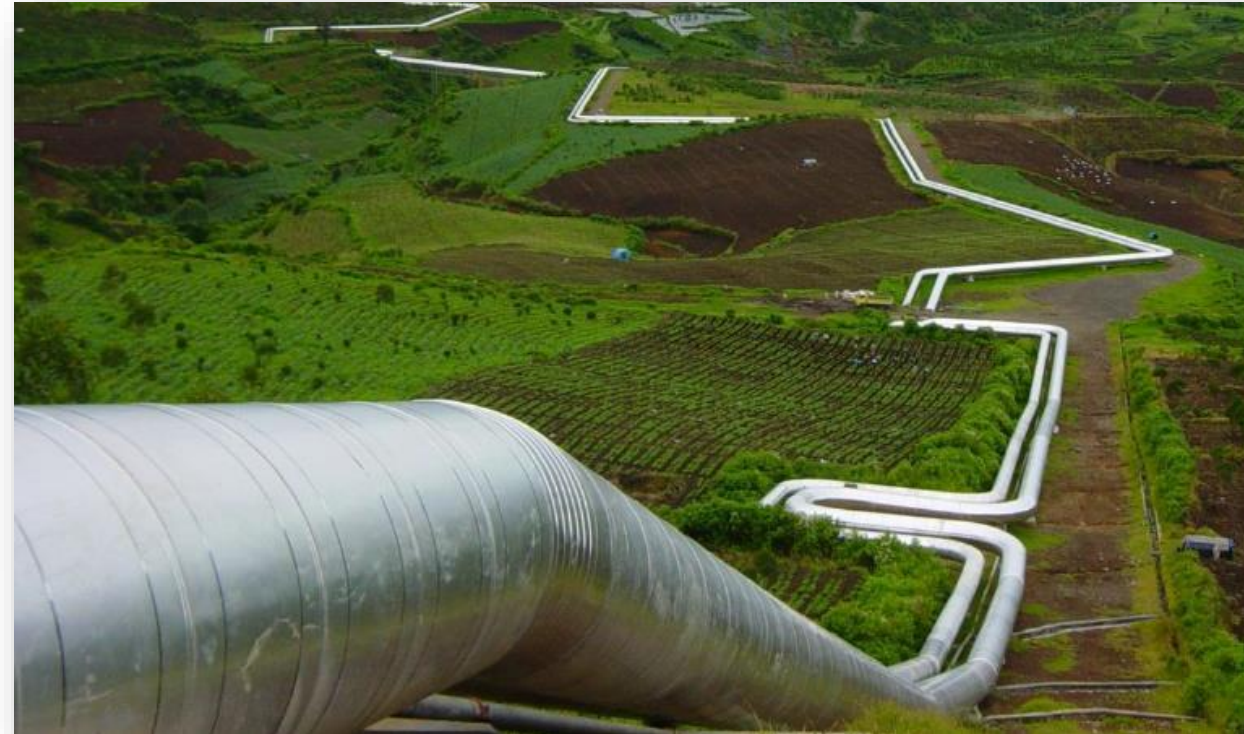
Two-phase pipelines in Wayang Windu
