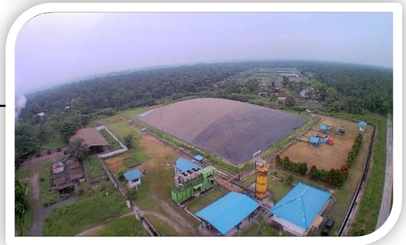
Biogas Plant Pagar Merbau 1 MW
